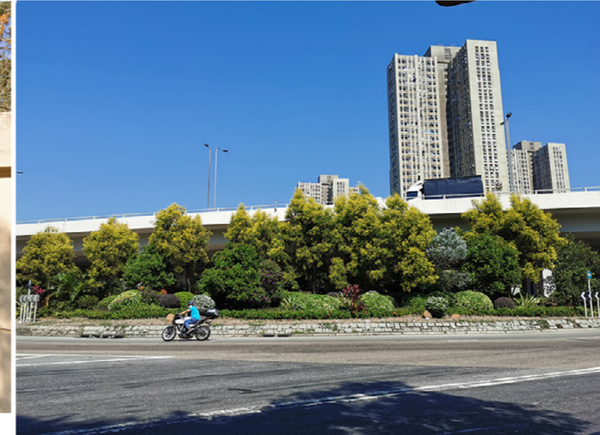
LR11.1 FANLING HIGHWAY
