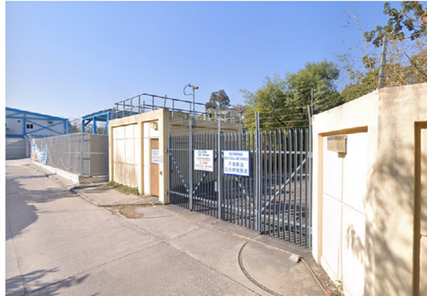
LR10 TOWNGAS OFFTAKE STATION, WATERWORK DEPOT AND OPEN STORAGE YARDS
